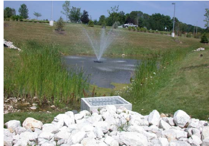
New developments require stormwater management such as ponds to hold and filter runoff.
