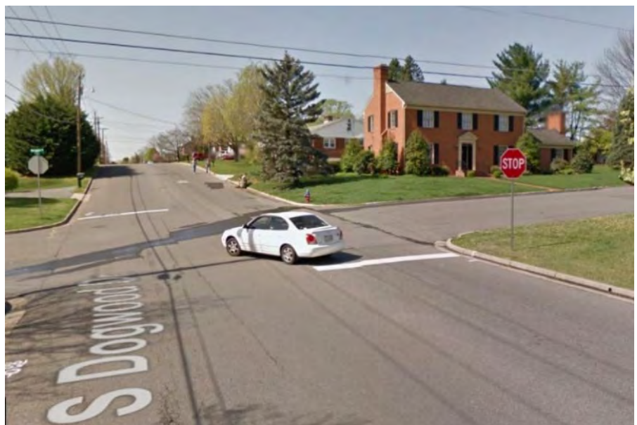
4) Stop bars at stop signs
