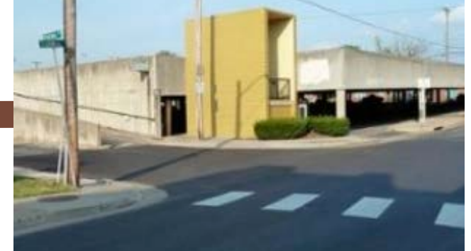
2013 – Parking deck built in 1971 on the corner of East Elizabeth and Federal Street
