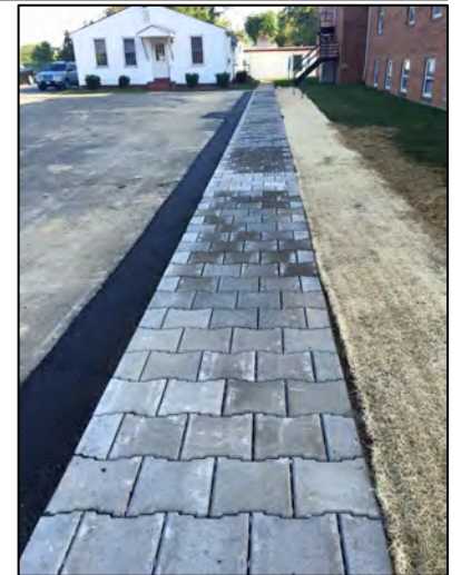
Below: Permeable pavement along parking lot
