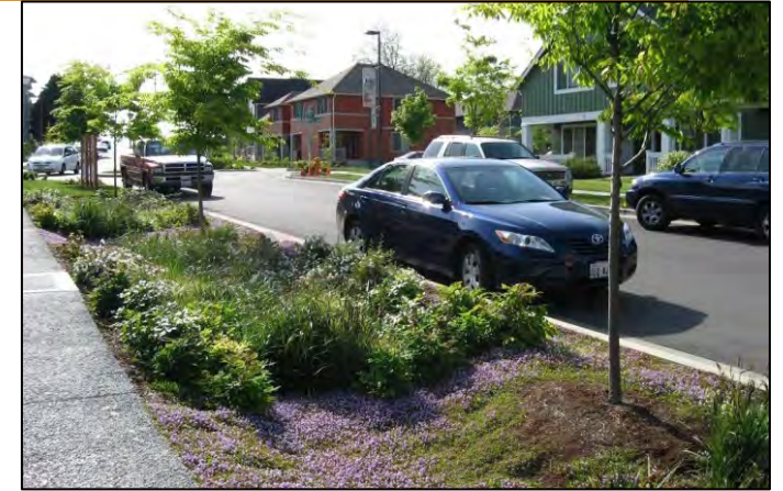
Above: Bioretention system in a right-of-way
