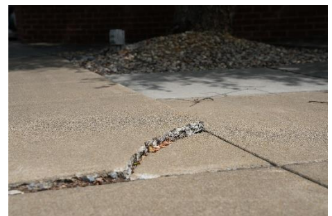
(Above) Existing river birch tree roots lift concrete and underground utilities in the Public Safety Building Plaza.
