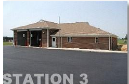
(Above) Fire Stations #2 and #3 now have working fire sprinklers thanks to a federal grant from FEMA.
