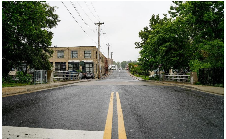
Crews will soon begin work on a bridge rehabilitation project on West Rock Street (above) near North Liberty Street as part of an ongoing series of such projects. Some temporary lane closures may take place during work, though roads will remain open to traffic.
