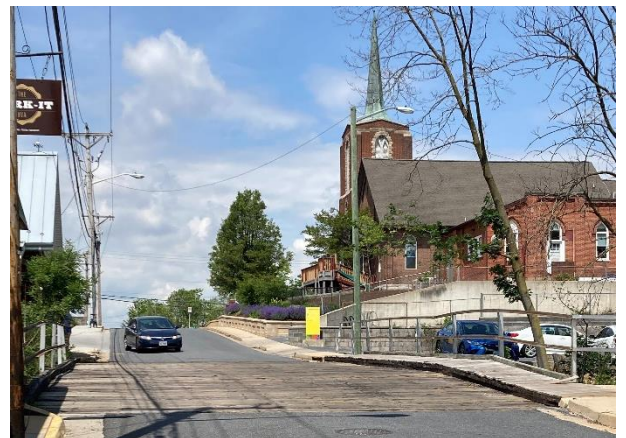
(Above) The West Water Street bridge over Norfolk Southern rail line. The bridge will be closed Wednesday.
