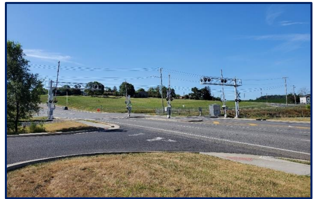
(Above) Norfolk Southern Railroad will conduct needed repairs to the Erickson Avenue railroad crossing next week.
