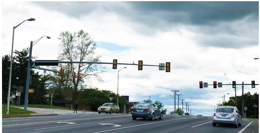
(Above) Work will improve the two South Main Street left-turn lanes onto Port Republic Road.
