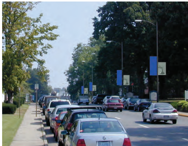
Retrofitted lighting along South Main Street.
