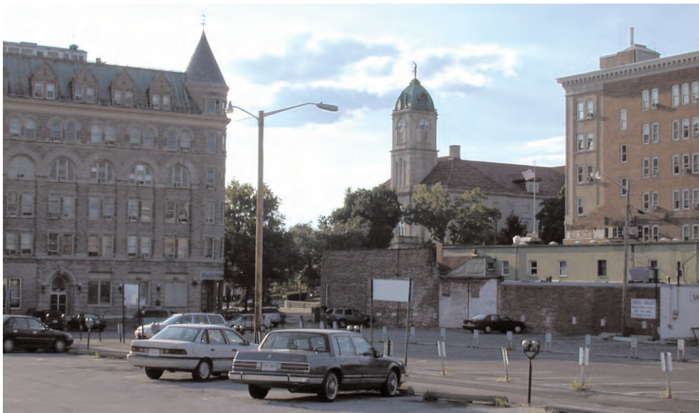
View of County Courthouse and Bank of America Building from Federal Street. The Post Urban Renewal and Downtown Core Districts offer tremendous potential for large scale mixed-use development.
