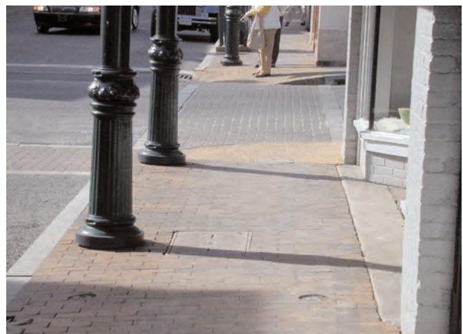
The streetscape plan replaces the checkerboard concrete pattern with a uniform running bond brick pattern replicating Harrisonburg’s 19th and early 20th century sidewalks, as shown in this image.
