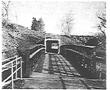
A tunnel constructed under a fill slope
