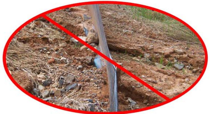
Silt fence shall be entrenched, backfilled and compacted.
