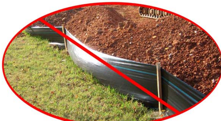
Sediment shall be removed from fabric.
