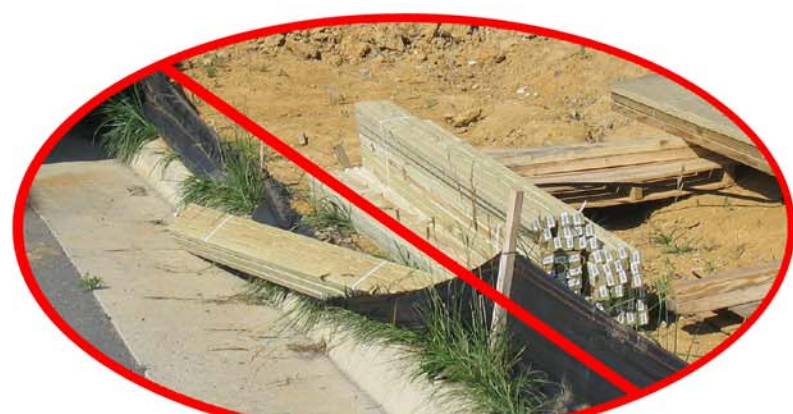
Damaged fabric shall be repaired or replaced immediately.
