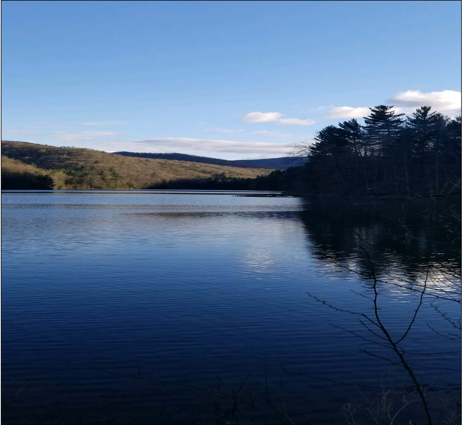
Reservoir at Switzer Dam
