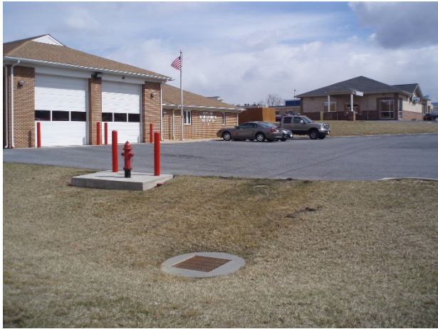
Figure 1: Existing inlet at edge of parking lot
