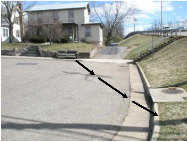
Figure 1: Dead end of Old South High Street. Block drainage inlets to force runoff towards camera.
