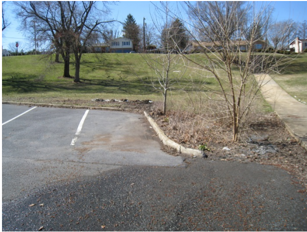
Figure 1: Small rain garden filled with grit and dirt Figure 2: Opposite view of rain garden and lot
