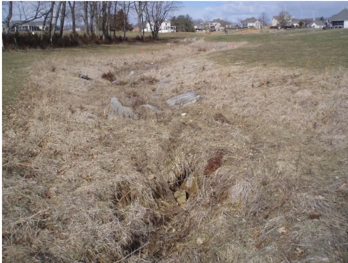
Figure 1: Eroded ditch below existing outfall in golf course
