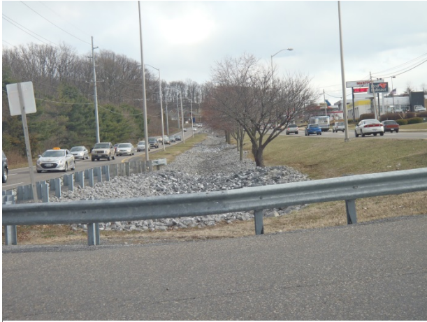
Figure 1: Rock-lined conveyance channel
