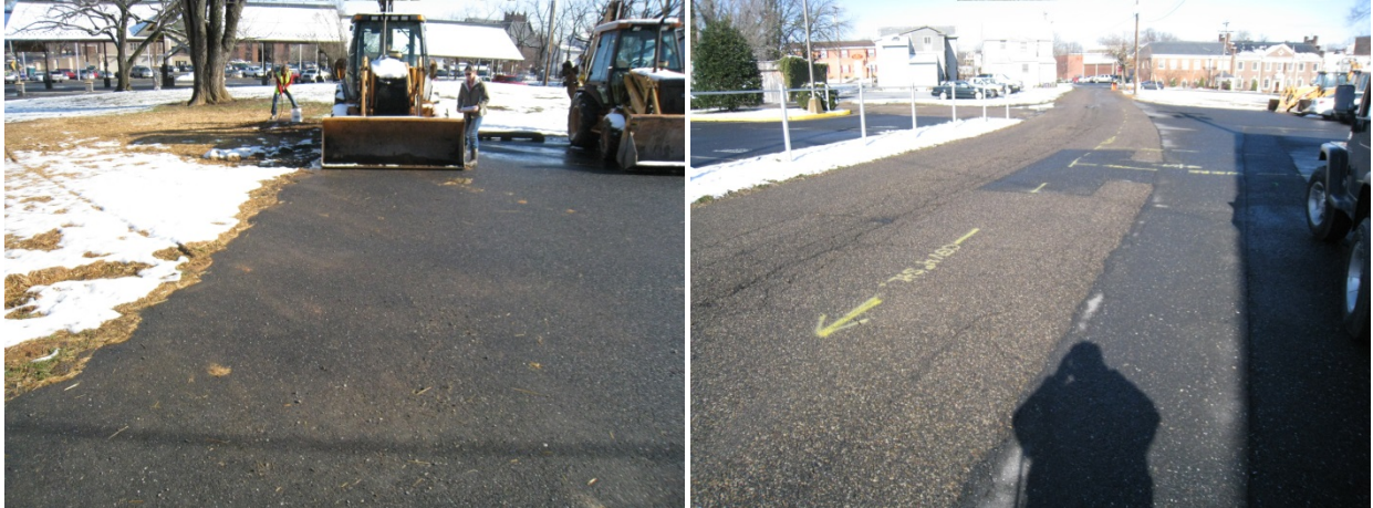
Figure 1: Bioswale can be located to left of asphalt Figure 2: Drainage area looking down Warren St.
