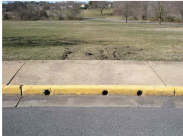
Figure 2: Existing drainage outlets to relieve ponding in parking lot
