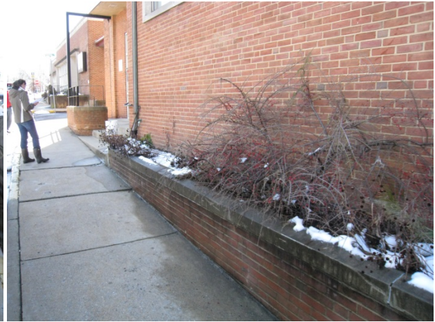
Figure 2: Existing planter bed
