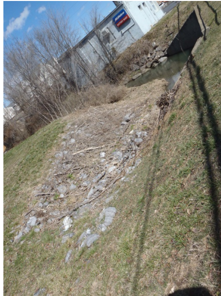
Figure 2: Rip-rap at downstream end of grass swale
