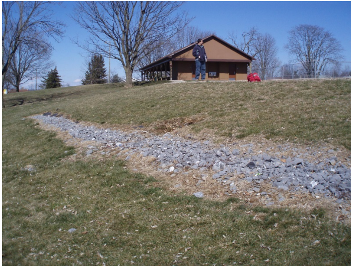
Figure 1: Existing level spreader below parking & travelway
