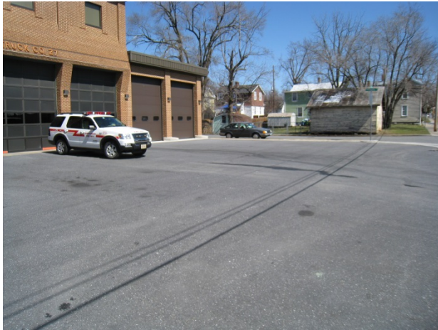
Figure 1: Stains on asphalt from wash water
