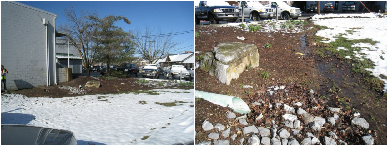
Figure 1: Small landscape area, N. side of building Figure 2: Roof drain outlet on left & eroded area
