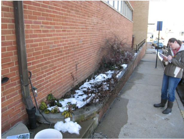
Figure 1: Downspout next to planter bed
