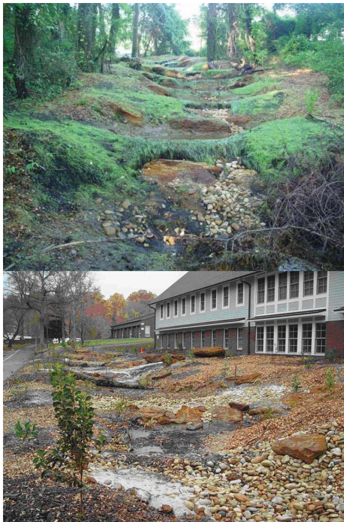
Figure 1. Examples of regenerative stormwater conveyance systems.
